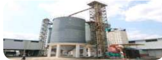
Storage facility (husk)
