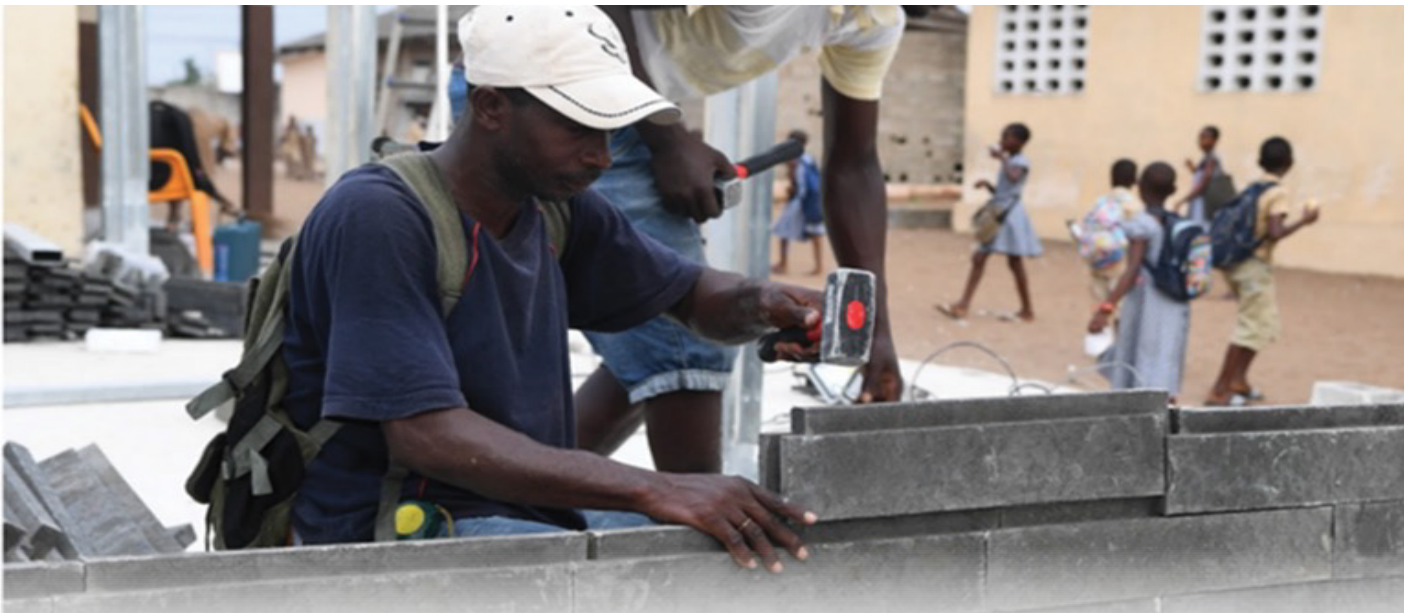
School construction using blocks made from recycled plastic
